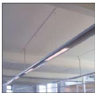
Figur 13: Eksponert betongdekke i kontorareal Foto: The Concrete Centre / The British Cement Association
