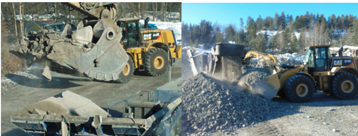
Fig. 1.1 Feeding of pre-stressed hollow core concrete rubble into an impact crusher (left) and the final product of 0/100 mm RCA (right), photo: SINTEF.
