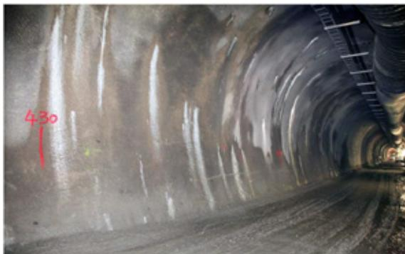
*Figure 1 - Tunnel wall sprayed with standard concrete (without polymer) during construction in 2008: visible water infiltration and white patches of discoloration caused by Ca(OH)<sub>2</sub>, etc. Similar observations were made during inspections in 2012 and 2018; never dried fully.*
