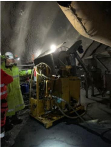
Figure 6 – Pump set-up for cement grouting
