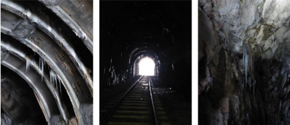
*Figure 1: Pictures of water penetrating the lining and creates icicles in an existing tunnel.*
