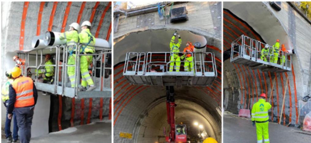
Figure 4: installation of the Mapeplan 3S membrane by adhesion with the Mapeplan Contact V fixing strips
