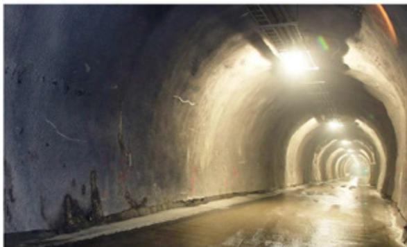
*Figure 2 - Tunnel wall sprayed with polymer-modified concrete during construction in 2008, 2 months after application: dry surface, no water migration.*
