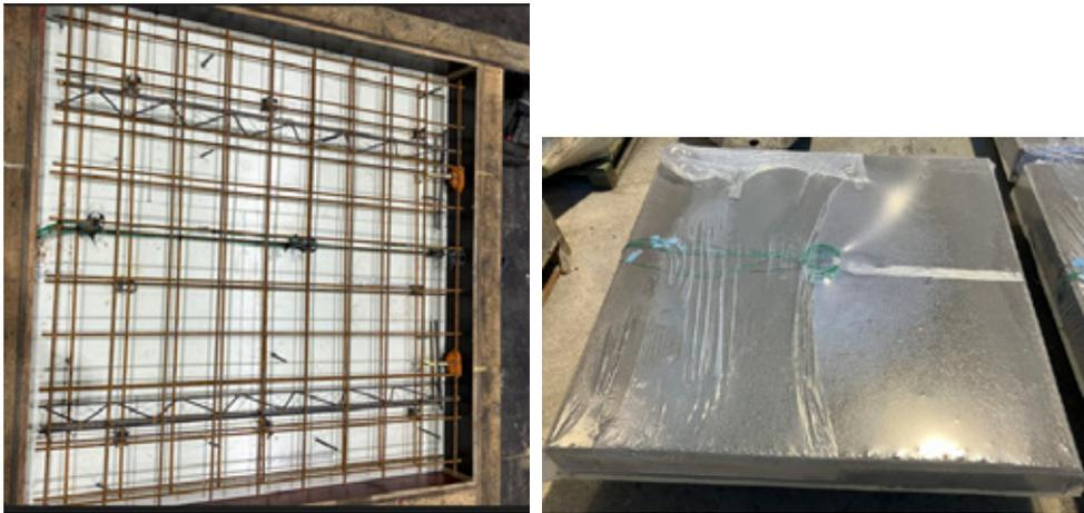
Figure 7 Formwork with two layers of mesh reinforcement, thermocouples and lifting anchors, ready for casting (left). Cast elements wrapped in plastic (right)
