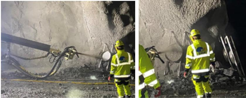
Picture 3 and 4: Moving the spraying nozzle sideways from wall and into the EATP-form, starting at the lower part. Then moving upwards and filling the EATP-form completely.
