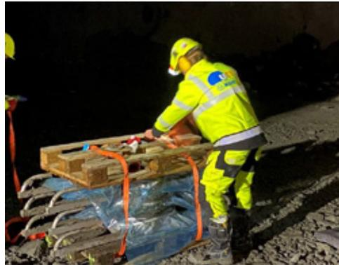
Picture 9 and 10: Placing three EATP-forms with sprayed concrete together in a “sandwich”, with pallet under and on top.
