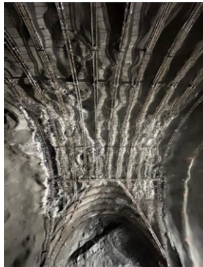
*Figure 4 Complex installation of lattice girders.*
