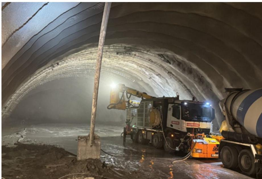
Figure 2 – AMW sprayed concrete equipment.
