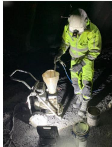
Figure 7 – Pump set-up for epoxy grouting.
