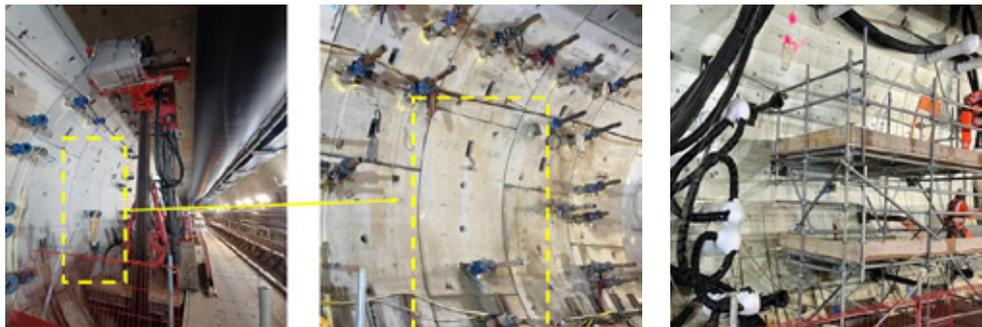
Figure 7 – Construction stages during CP AGF construction; drill rig setup (LHS), CP opening (Middle), segment coring (RHS)
