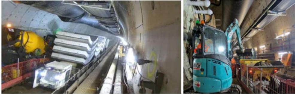
*Figure 10 – MSV travelling at a CP platform (LHS), SCL muck away (RHS)*
