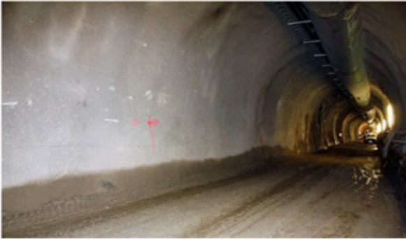
*Figure 3 - Inspection of the tunnel wall sprayed with polymer-modified concrete at 480 m: waterproof during the first inspection in 2012 and the latest inspection in 2018; dry surface.*
