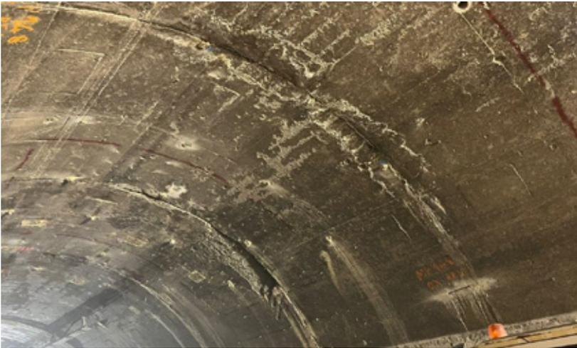
*Figure 2: state of degradation of the "Manfreida" tunnel.*
