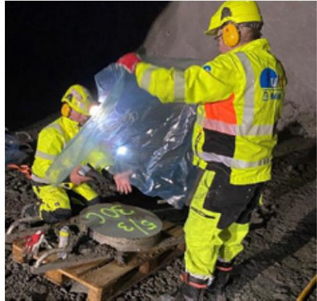
Picture 7 and 8: Scraping off remaining concrete (thicker than 100 mm) and marking and wrapping in sample with plastic sheet.
