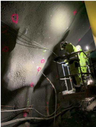
*Figure 3 – Void filling with cement grout.*
