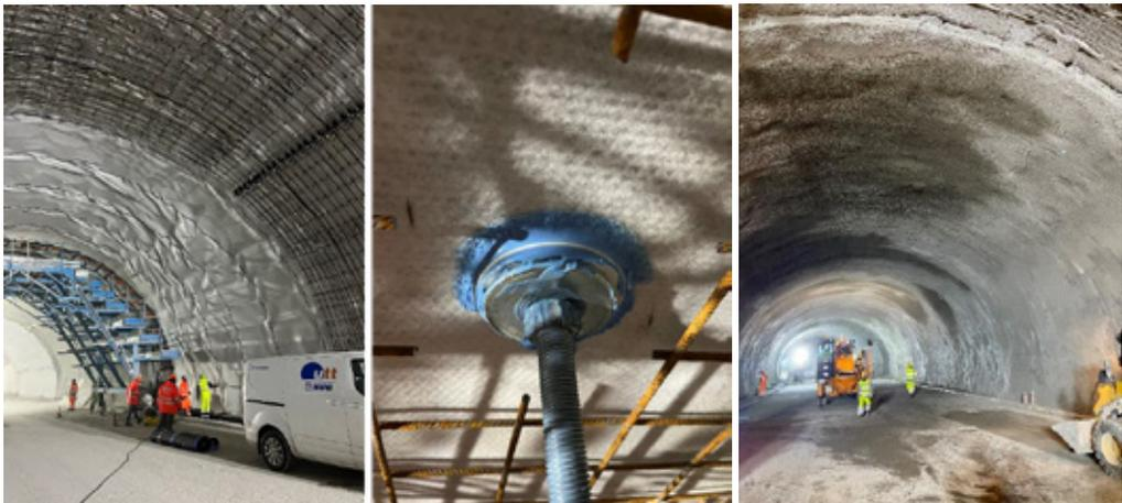
Figure 6: completely installed waterproofing layer and rebar arches (left), detail of structural connection passing through the waterproofing layer (center), completed shotcrete lining in the Manfredia Tunnel (right).
